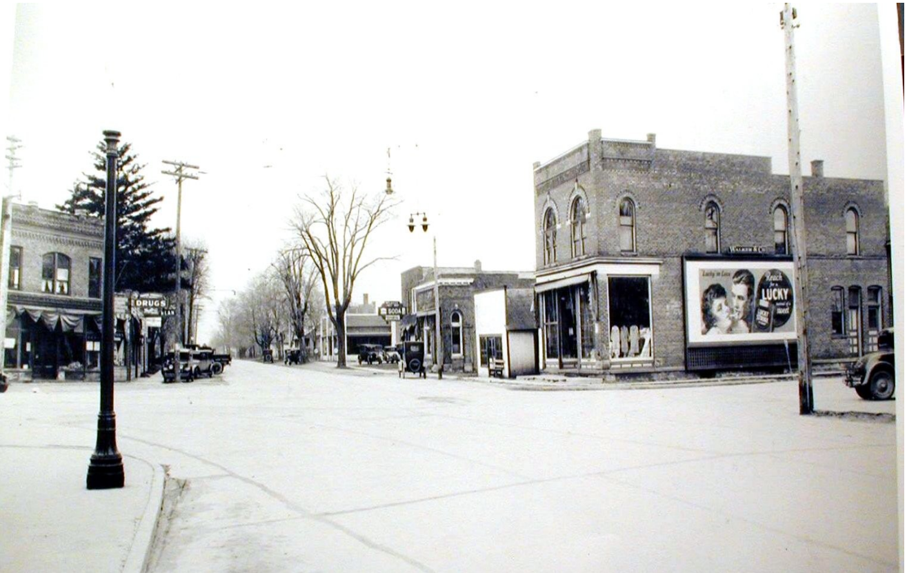
Great foto showing Moore and Peck corners electric street lighting guess early 1930s
